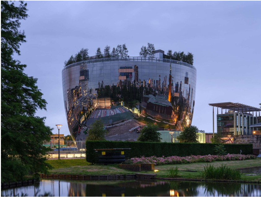
Depot Boijmans van Beuningen, MVRDV 2021, with roof garden, Rotterdam
